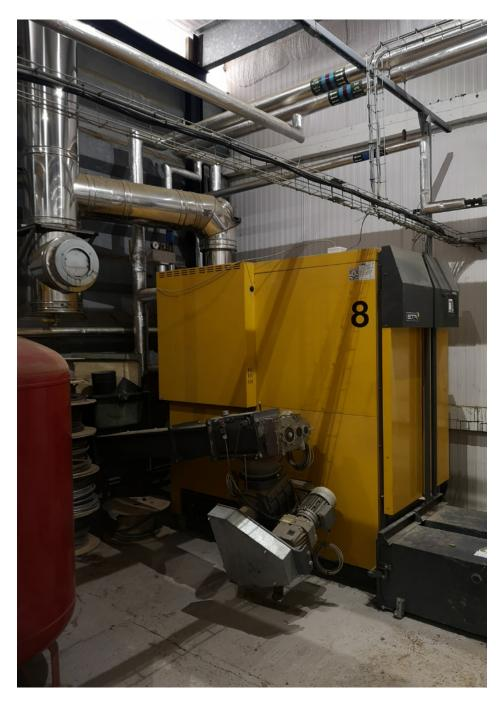
This shows how the wood chips feed into the machines
