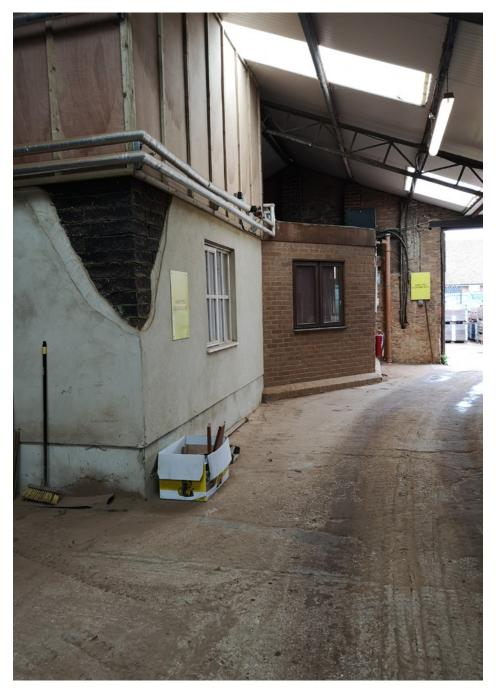
Entrance into main brick making area. This is a view of the offices. The office on the end is intentionally peeling away the wall to show the construction of their strocks and mortar work.
